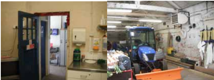
The old locker room and (right) where the old boilers once stood
