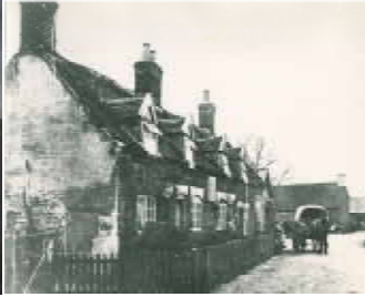
The former Tablet Cottages and the tablet that is now located on the front wall of Rushmere Baptist Chapel
